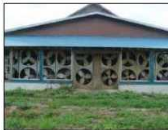
↑牛舎壁面の換気扇
