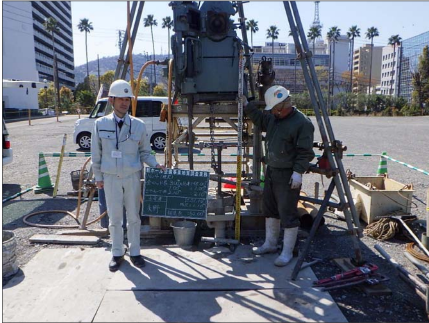
No. 4 削孔長検尺
