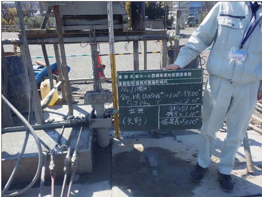
No. 1 削孔長検尺
