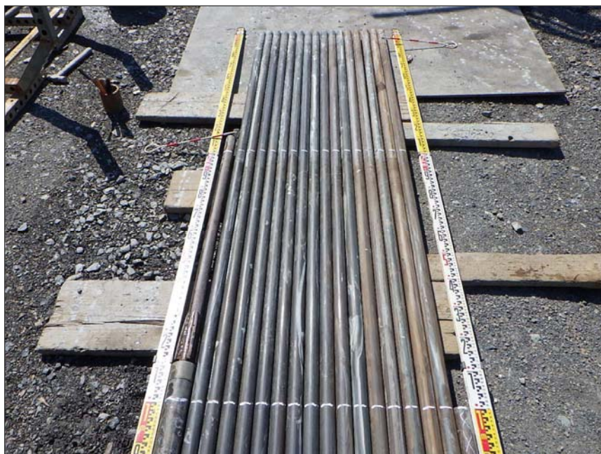
No. 4 削孔長検尺
