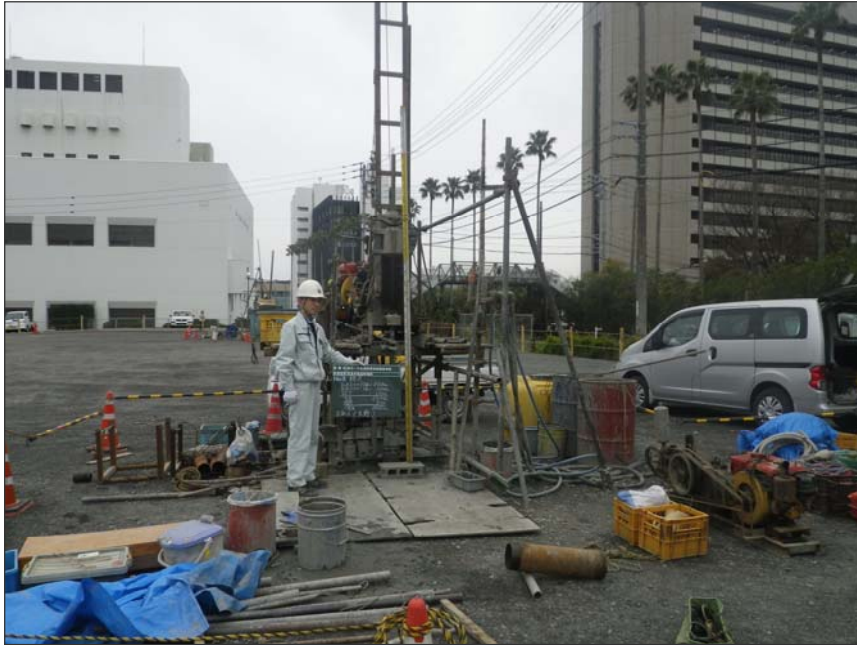
No. 3 削孔長検尺
