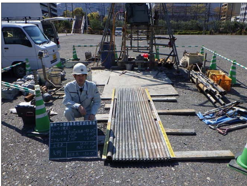
No. 4 削孔長検尺
