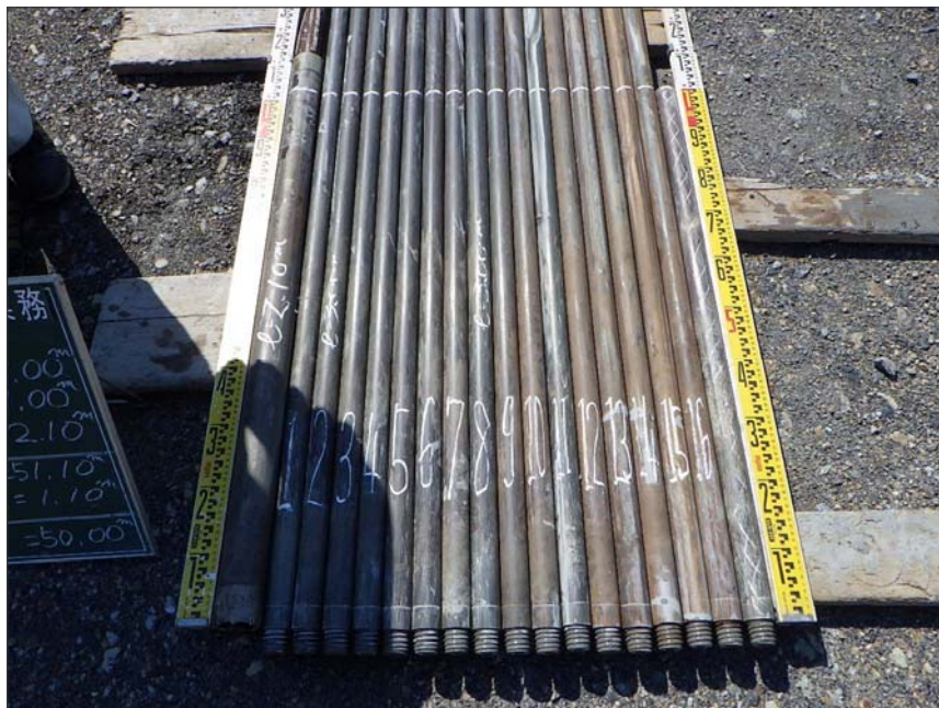
No. 4 削孔長検尺
