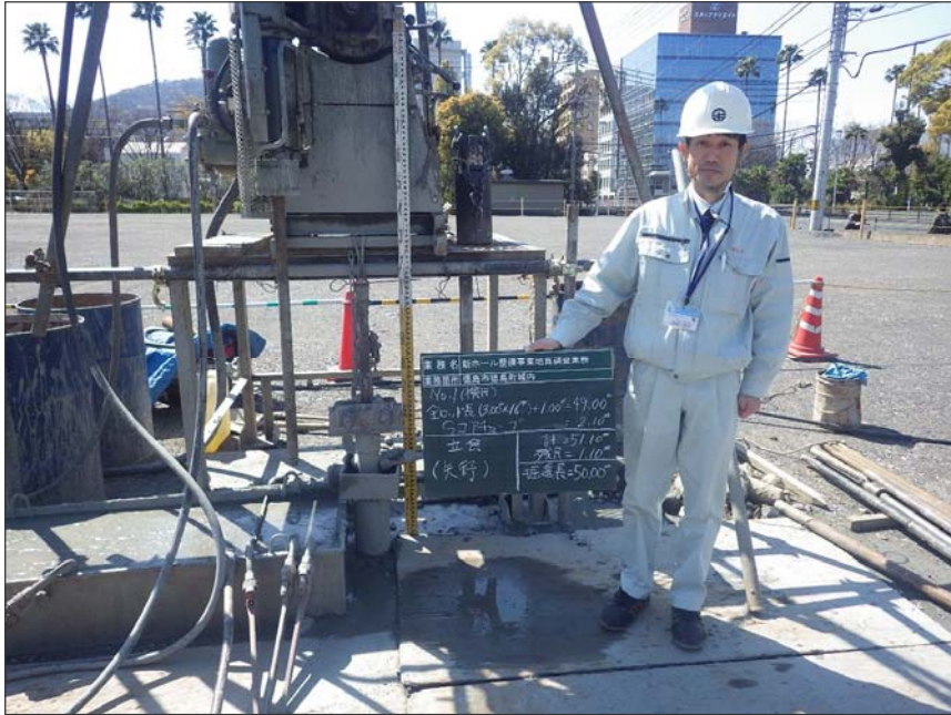
No. 1 削孔長検尺
