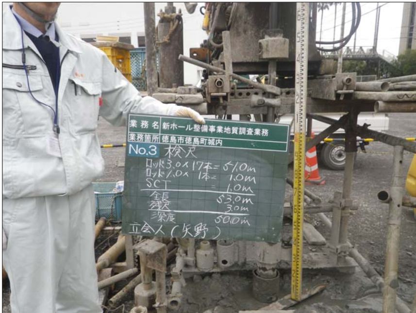
No. 3 削孔長検尺
