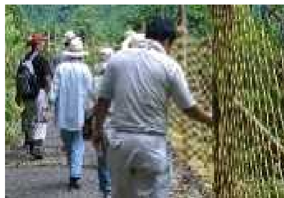
侵入防止柵の点検
