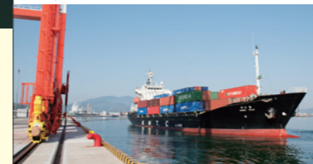
-10m岸壁 Quay water depth 10m
